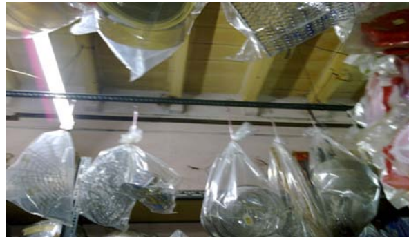
Fig. 23: Photograph of the first floor's timber floor on No. 16, Jalan Besar (left).
