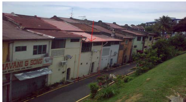
Fig. 32: Photograph of the roof and chimney found on No. 5, Jalan Besar.
