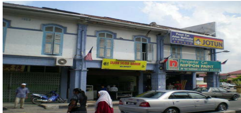
Fig. 4: Front elevation of the Early Shop house Style found in Jasin.
