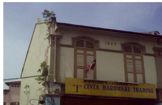
Fig. 22: Casement windows on the first floor façade of No. 16.
