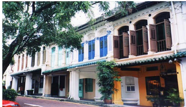
Fig. 34: Shop house in Emerald Hill, Singapore (right).
