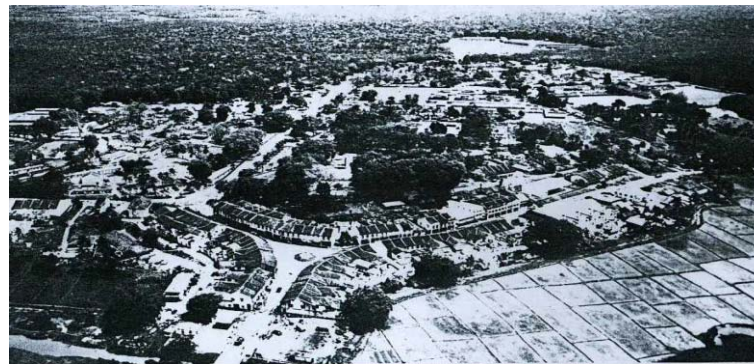
Fig. 1: Aerial view of Jasin Town in the 70's.
