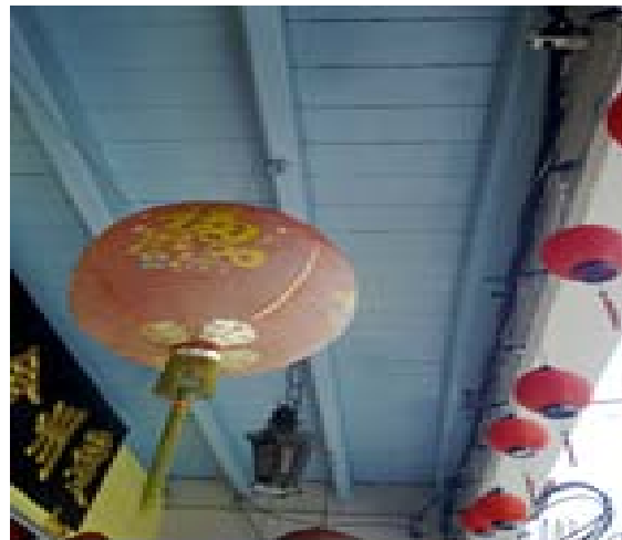
Fig. 31: Photograph of the hardwood floor joists crossing the span of the party walls at the walkway of No.26.
